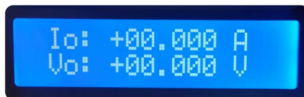
Figure 8: local display with current and output voltage monitor
